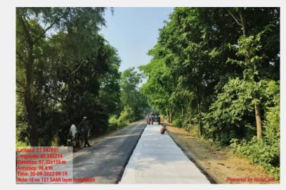
Laying of Paving fabric and Providing BC / PQC over the stabilized Layer
