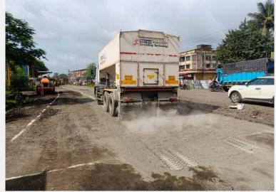
Cement Spreading by **Microprocessor Controlled** Spreader Truck
